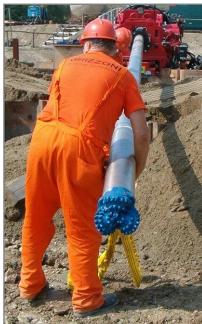
Figure 5.6 Bottom Hole Assembly
