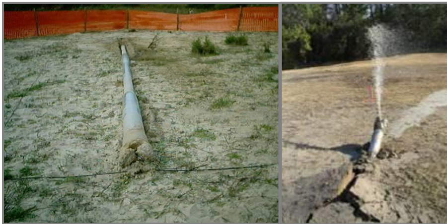
Figure 5.8 Completion of pilot bore hole... Exit Point
