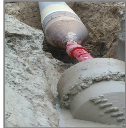
Figure 5.19 Pull back assembly: pipeline.
