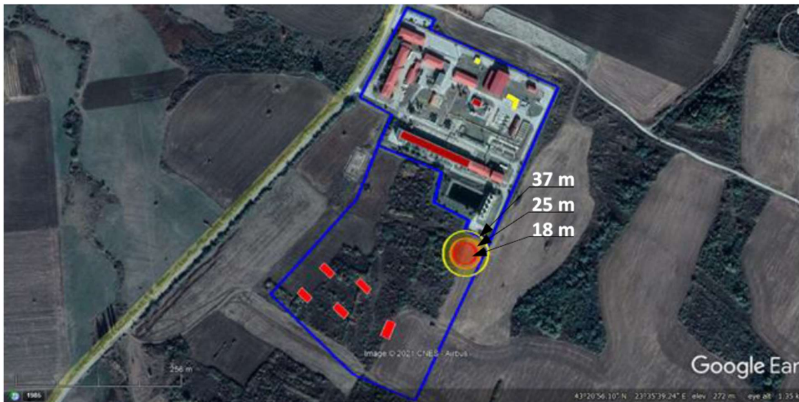
Figure II.3.2-9 Puddle fire in a tank storing 23.7 t of methanol
