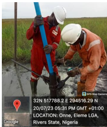
Figure 2.4: Installation of 2-inches casing pipes in GW3 Borehole
