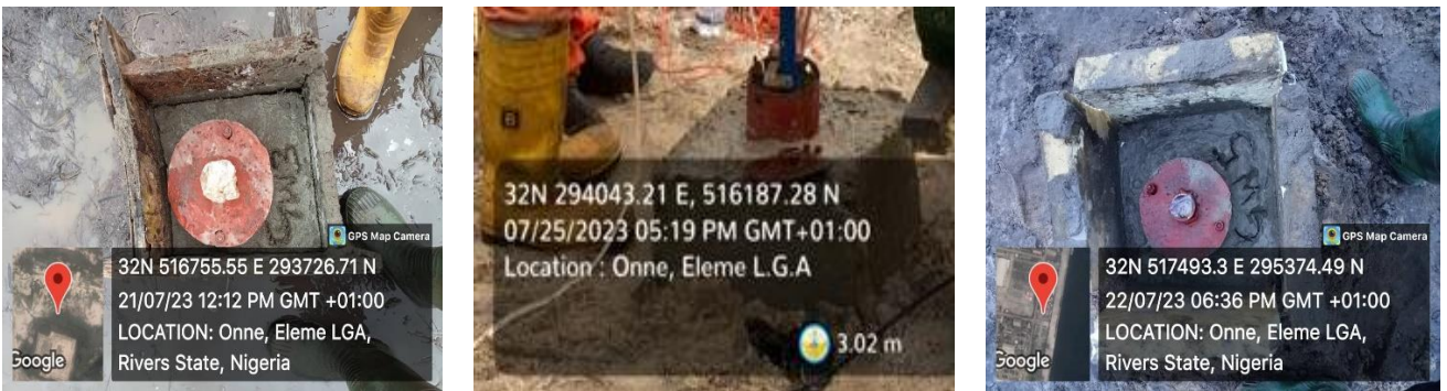
Figure 2.5: Well head installation for GW3, GW4 and GW5 boreholes
