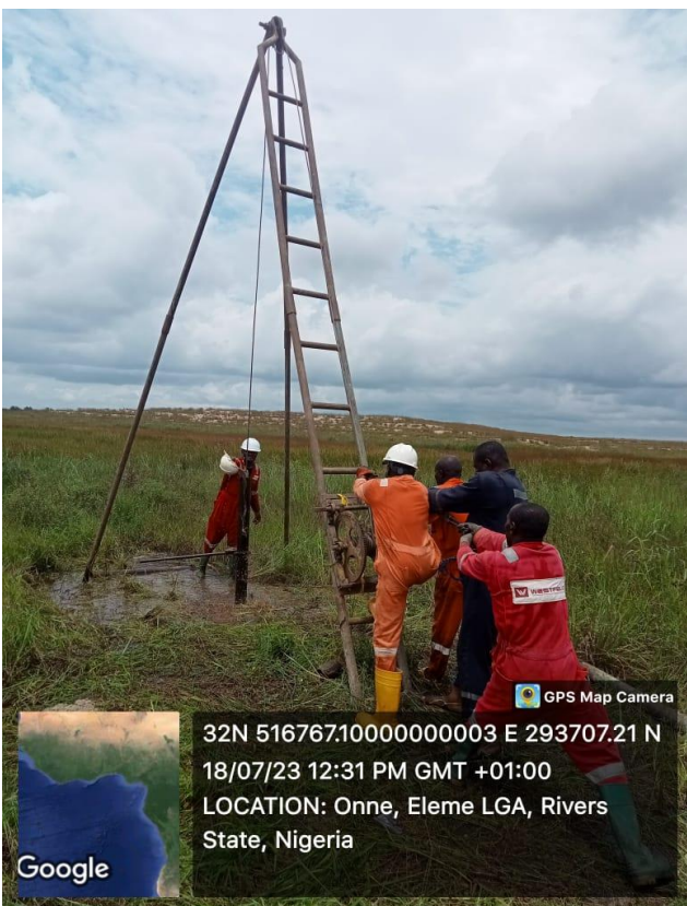
Figure 2.2: Drilling process using the percussion rig.
