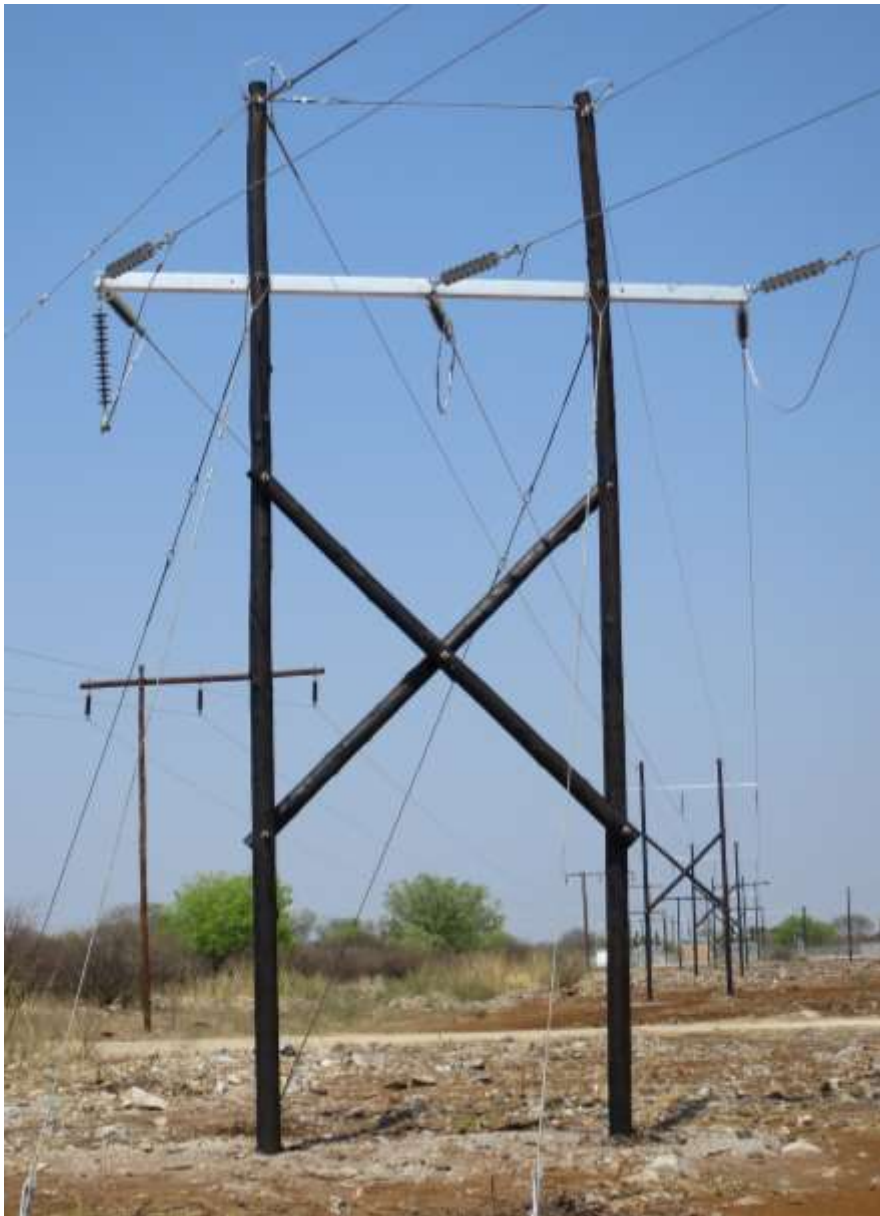
Plate 2.2: Example of the 66kV wooden structure with steel crossarm (Source: Transmission Consulting Services (TCS), 2020).
